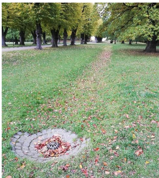
Figur 13. Svackdike i park.
